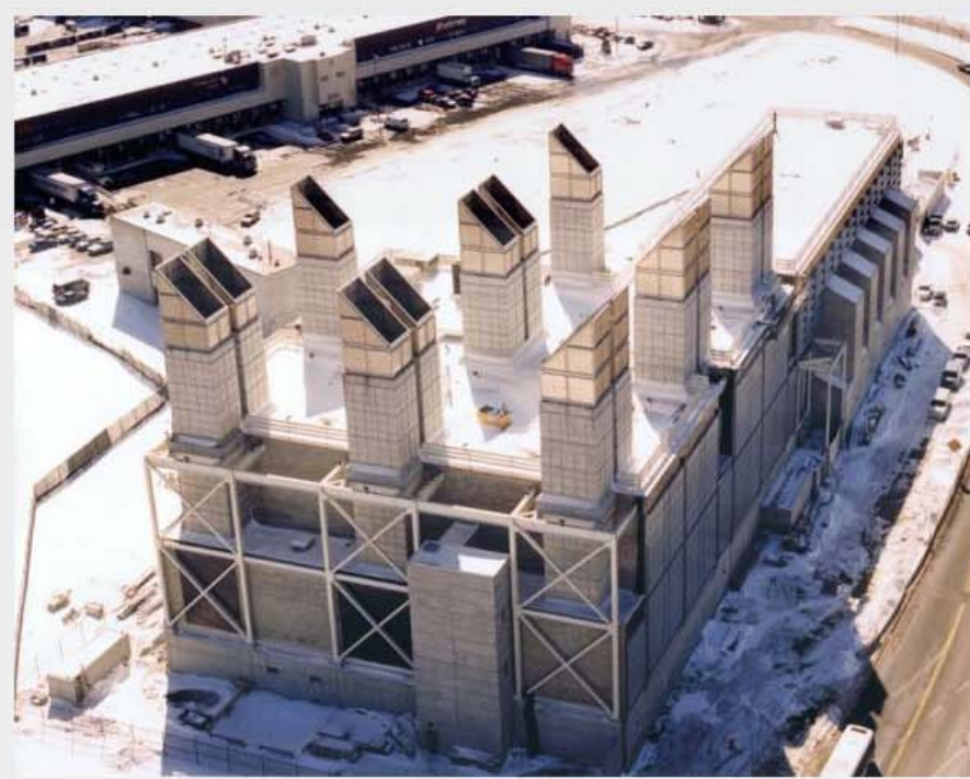
Central Artery Tunnel Ventilation Building No. 7 (Credit: Ryan Iron Works, Inc.)
