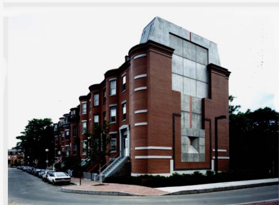
MBTA's Vent Building on Yarmouth Street
